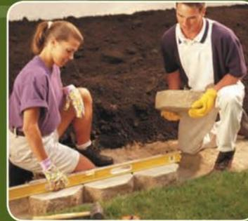
Place and level the first Keystone Garden Wall unit. Level each additional unit on the base course as you place it, making sure that the outside edges touch. If your wall contains both straight and curved areas, start with a straight area and build into the curves. Complete the base course before proceeding to the second course.
