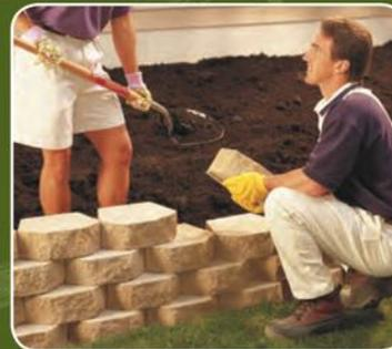
Starting with straight areas first, begin placing the second course. Center each Keystone Garden Wall unit on the seams of the course below in a running bond pattern as shown. Now proceed to the next layer, backfilling as you go. For drainage behind the wall, clean gravel or crushed stone is recommended.
