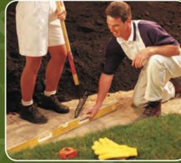
Start by digging a shallow trench 4" deep by 12" wide. Cut through and remove any sod, roots or large rocks. For organic loam soils, dig 4" deeper and add a leveling pad of sand or gravel. Compact and level the soil to receive the first course of Keystone Garden Wall.
