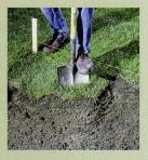
slope for correct water runoff. Slope can be in more than one direction depending on jobsite circumstances. Water will not penetrate joints unless it is allowed to puddle or remain in an area. Remove any loose soils after excavation is complete.
