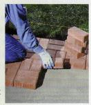
and final compaction is done. Slight adjusting can be accomplished by moving pavers to desired spot by inserting a flat head screwdriver in between pavers and pushing them. Cut pavers can be used to fill any voids in the pattern along the edges. Be sure to mix pavers from multiple pallets to achieve a consistent color
