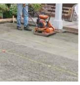
Base rock should have a certain amount of moisture content. Repeat steps until final base elevation is achieved. For a standard 1 <sup>3</sup>/<sub>4</sub>" architectural slab, the final base elevation should be 2 <sup>1</sup>/<sub>2</sub>" below final pavement elevation. Remember, the final product will mirror the base elevation. Any deviation in base should be corrected at this time with base rock (not sand).
