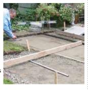
approximately 1" of sand screeded between the two pipes. Pull pipes out of sand; fill pipe voids with sand and trowel smooth. Do not compact sand bed.
